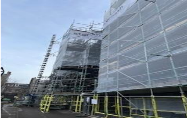
Phase 2 scaffolding ongoing
